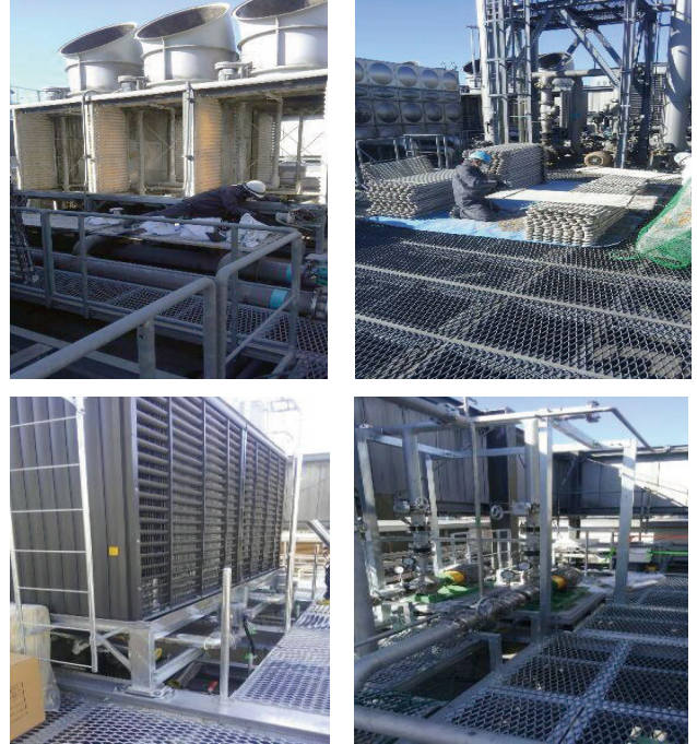
Fig. 1. Photographs of the four systems of RIBF cooling tower overhaul and new cooling systems for RILAC's superconductive.
