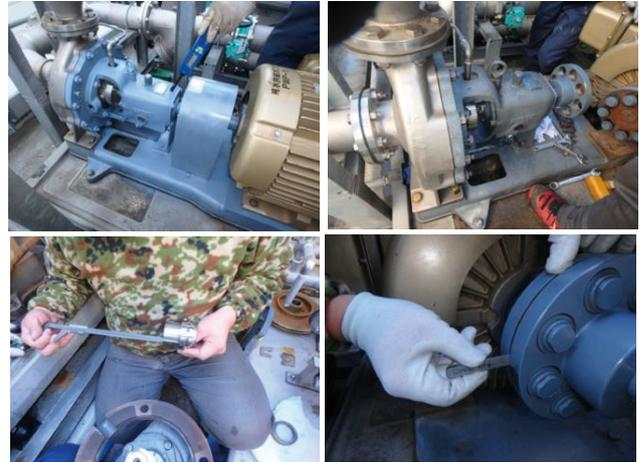
Fig. 1. Photograph of the RIBF Cooling water pump maintenance.
